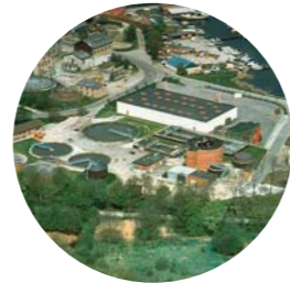
Hobro, Denmark (1994) Nitrification/denitrification after physical-chemical settling. 6 cells, 28 m 2 each 75 000 PE
