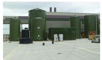
cutting edge renewable energy opportunities. Accordingly low strength wastewater and grey water is treated in a reverse osmosis plant and recycled to the dairy for CIP. The biogas generated by the process is used to fuel the on-site CHP plant, helping Arla in its aim to be carbon neutral.
