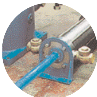
Hydraulically linked chemical dosing cylinder
