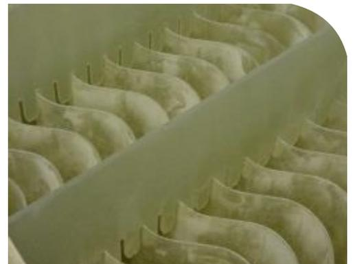
Figure 2.1 Left: The fine bubbles created by Dissolved Air Flotation. Right: GRP plate pack
