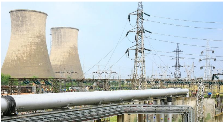
Power plant at Ploesti Dalkia Rumania. Source: Photothèque VEOLIA - Manolo Mylonas
